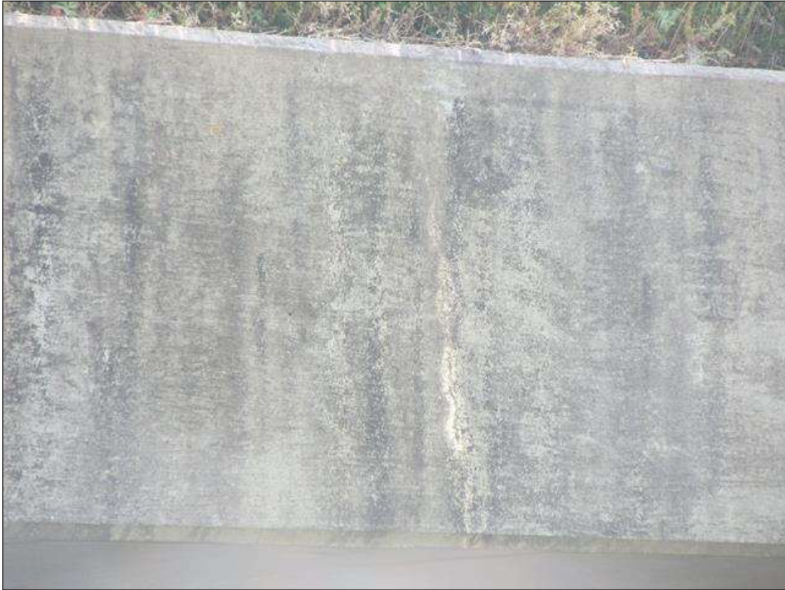
CRACKS IN BOTH HEADWALLS
