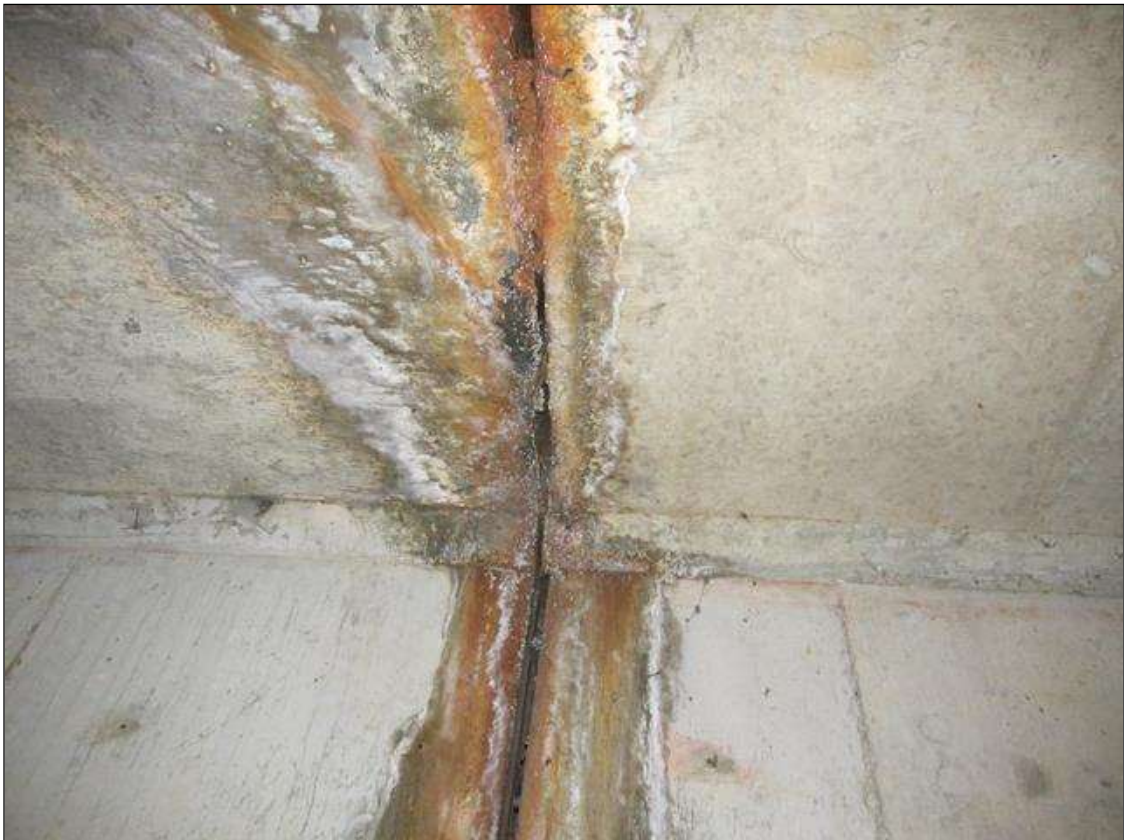
OPEN CONSTRUCTION JOINTS
