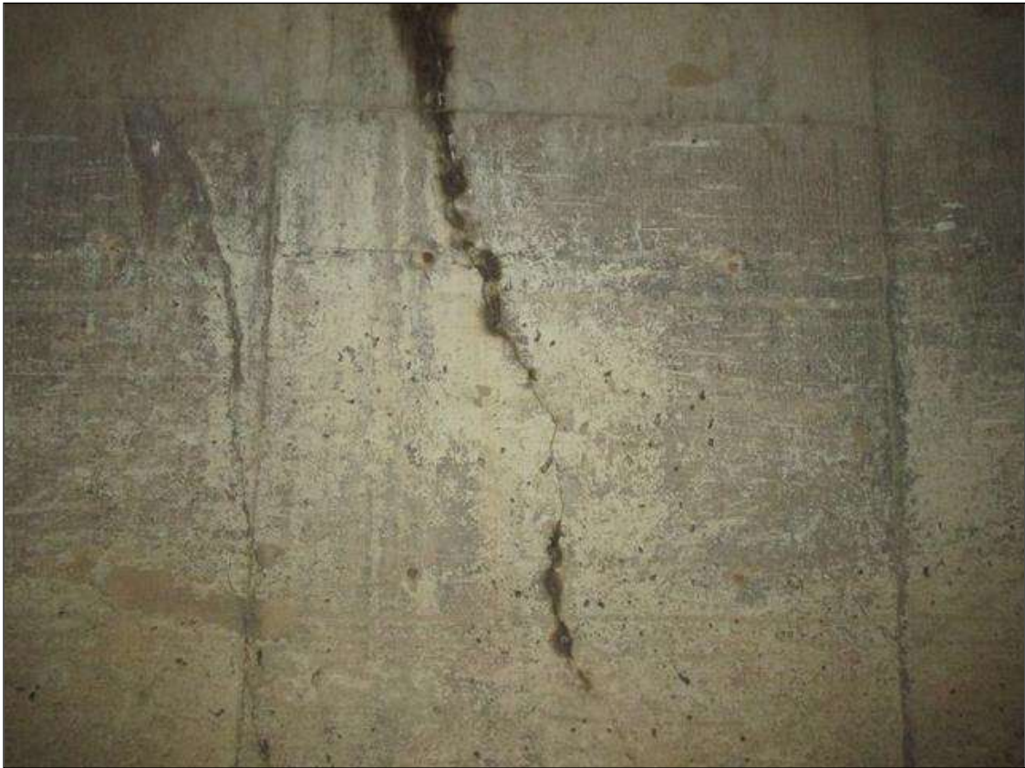
CRACKS IN ALL WALLS
