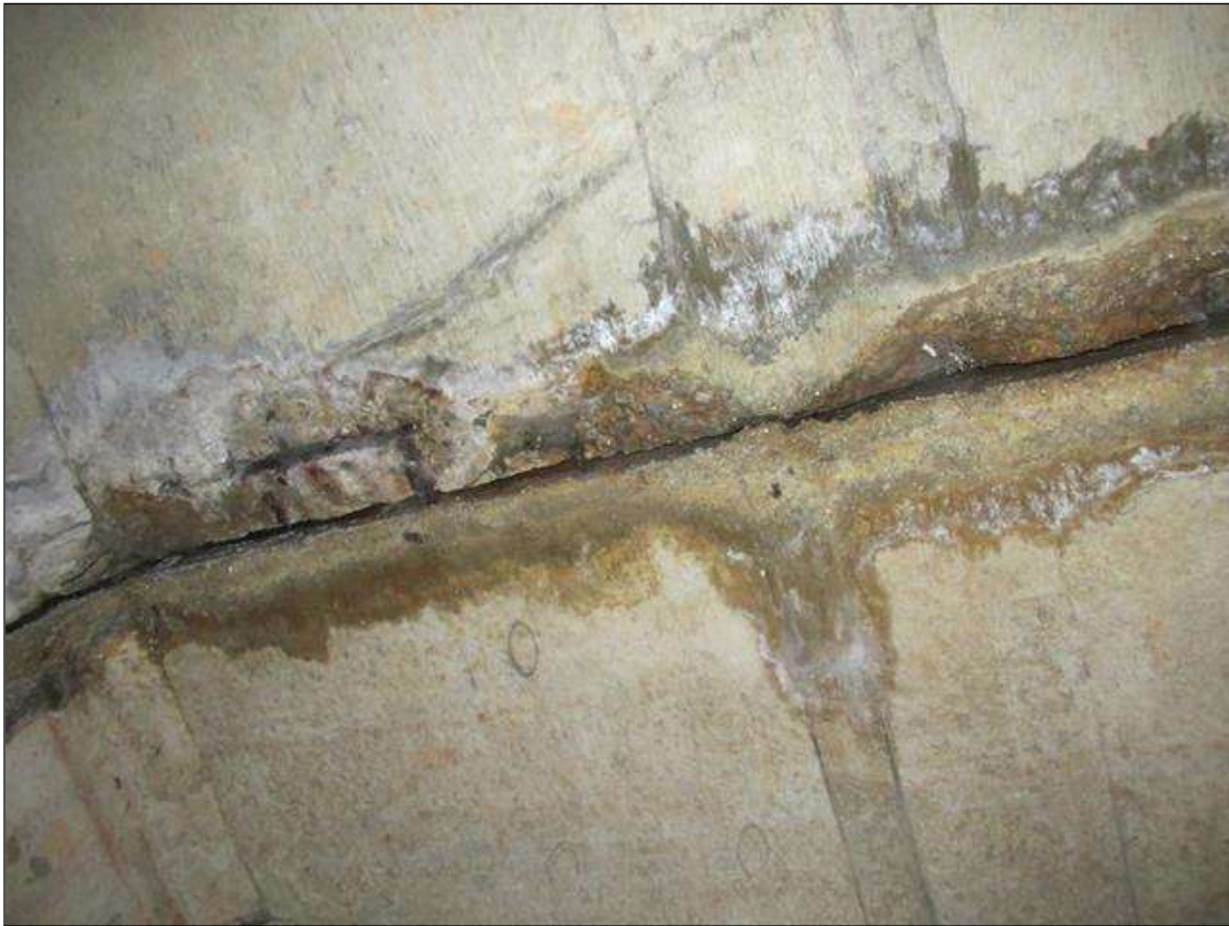
SPALLS ON THE TOP SLAB 80 FT. FROM THE INLET END WITH REBAR EXPOSED
