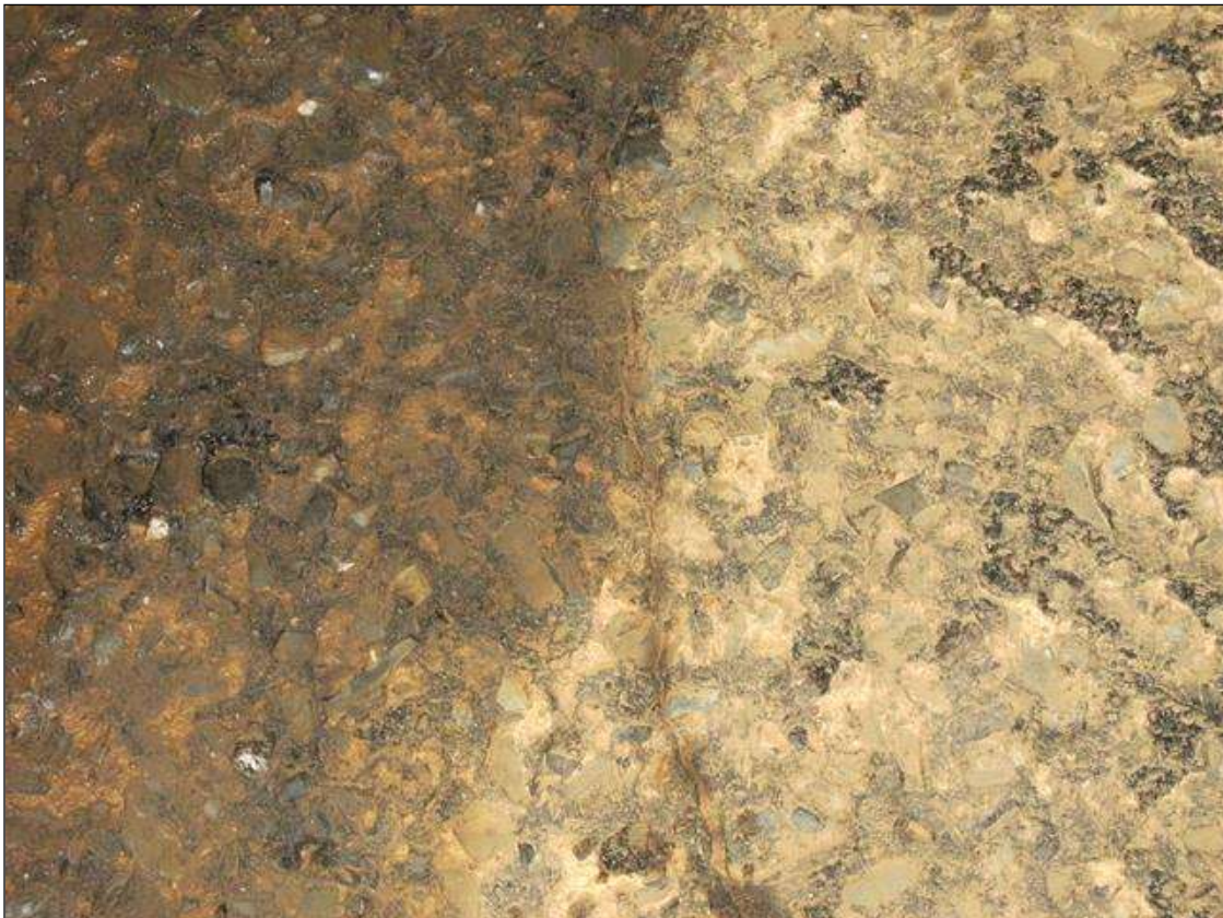
LONGT. CRACKS IN THE BOTTOM SLAB OF BARREL 2 UP TO 1/16" WIDE
