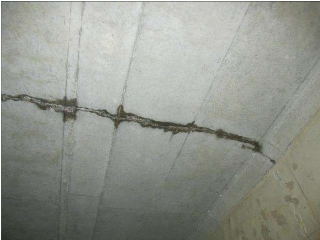
CRACKS IN THE TOP SLAB
