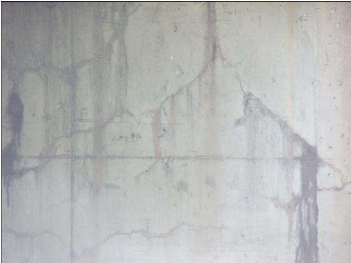
HL. MAP CRACKS IN EXTERIOR WALL # 2, LEFT END
